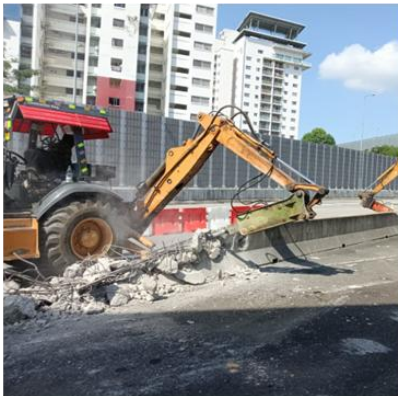
Installation of Emergency Median Opening
