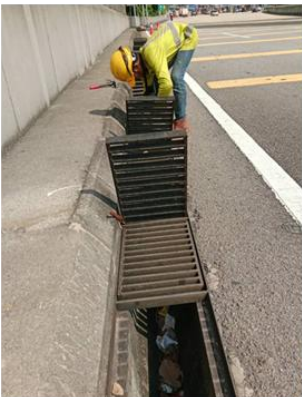
Drainage Cleaning
