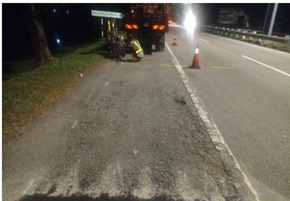
Pothole Repair
