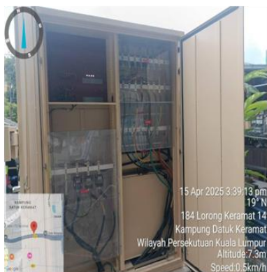
Replacement of Rusty Street Lighting Main Feeder Pillar
