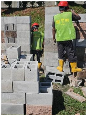
Installation of Noise Barrier
