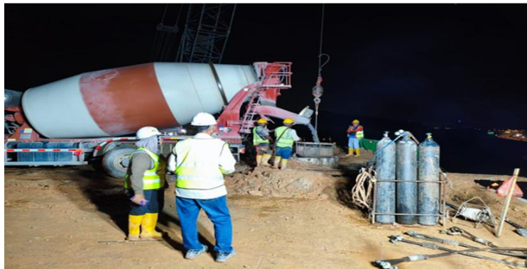
Concreting works at Abutment B
