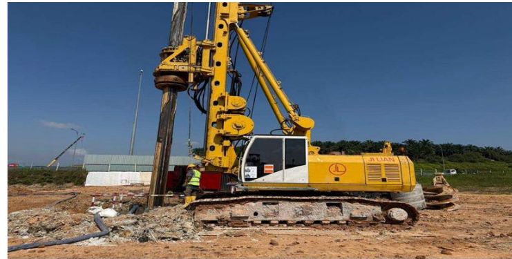
Bored piling works at Pier 6
