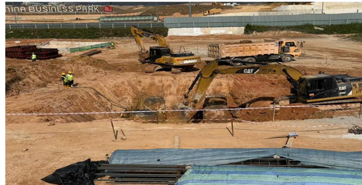
Excavation work pile cap Pier 6
