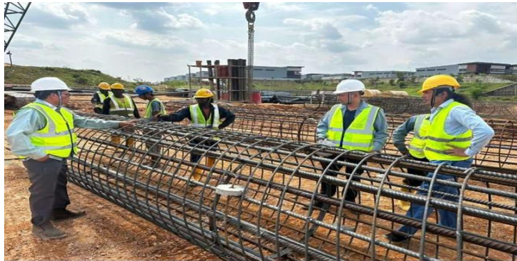
Rebar cage for bored pile inspection by Consultant
